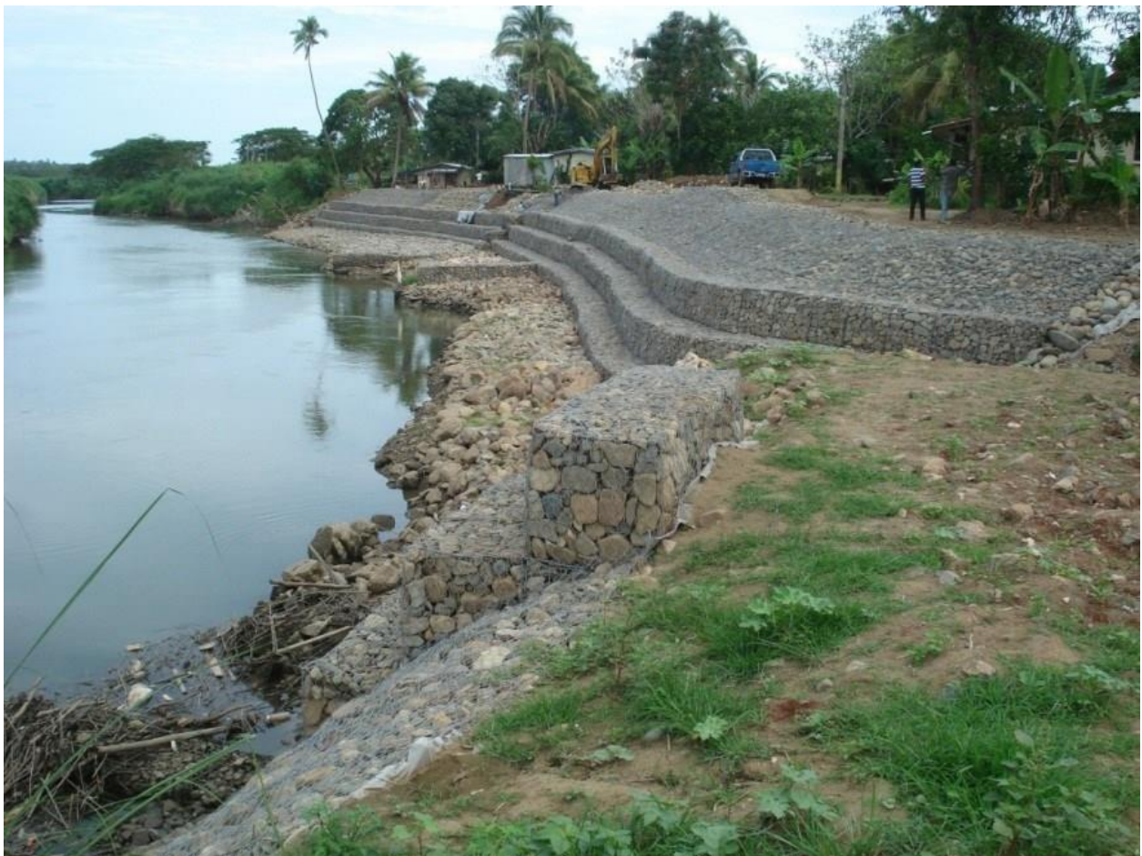
Figure 4: Construction of gabio Groynes at Narewa Village in Nadi (source: https://mwlfiji.com/projects/ )
