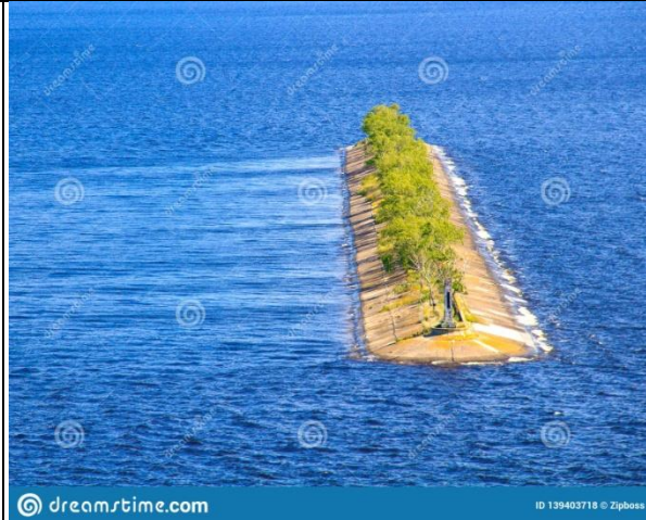
A long concrete breakwater with green trees with waves on a bright summer day
