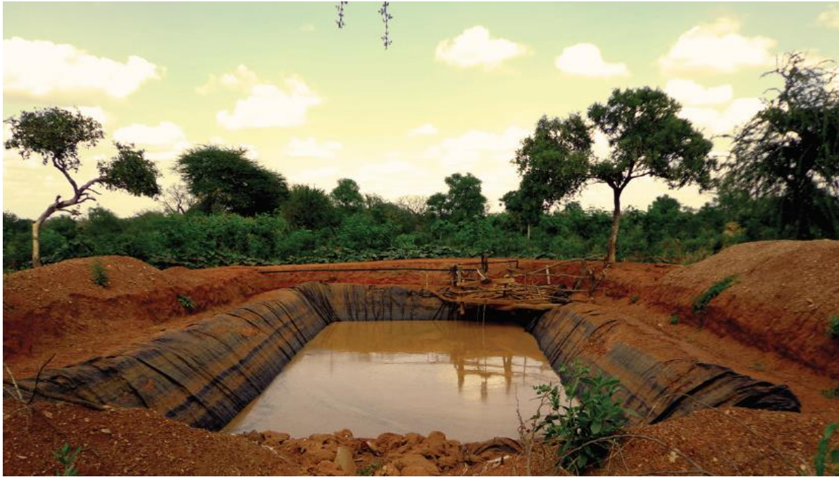
Figure 8. Surface rainwater harvesting
