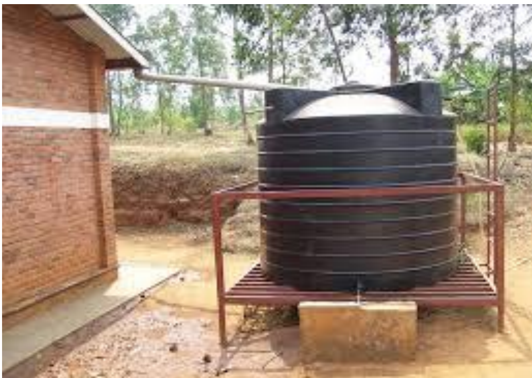
Figure 7. Rooftop rainwater harvesting
