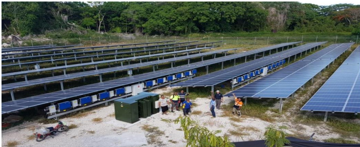
Figure 3: A 500 kW grid-connected solar farm in Nauru
