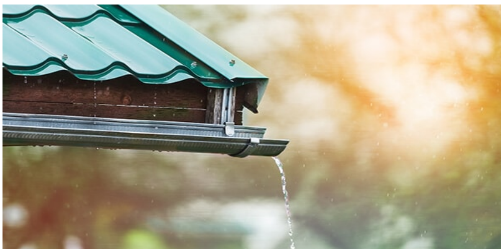
Figure 8: Rooftop rainwater harvesting system
