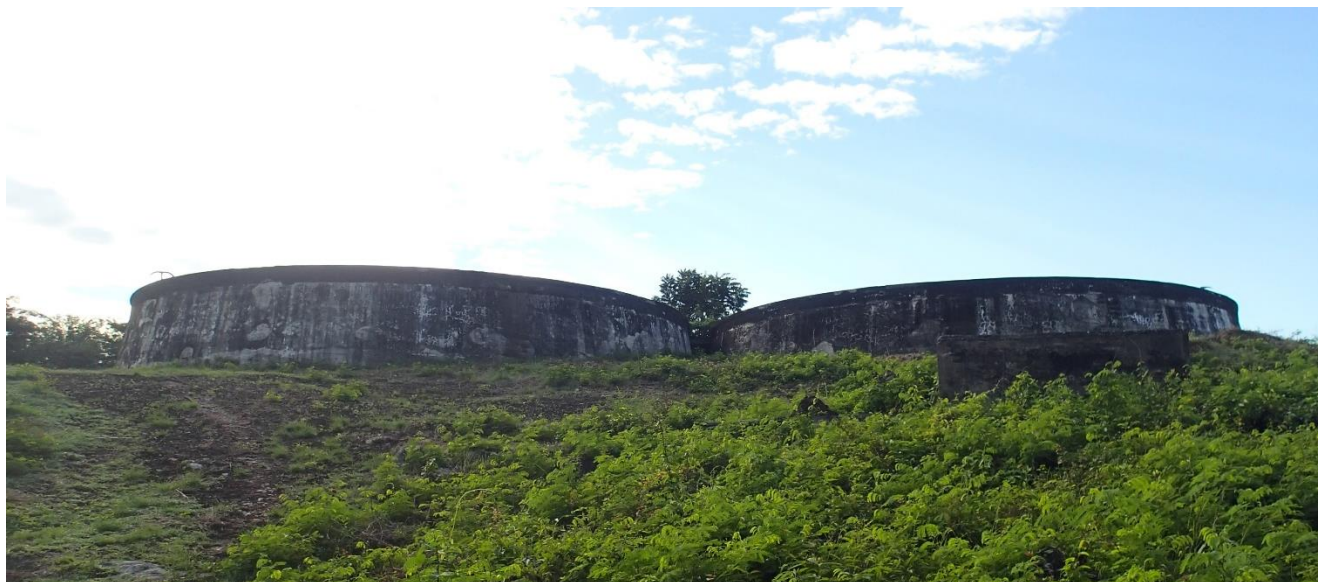
Figure 4-2: Large storage tank in Northern Clarendon used for the collection of water and distribution to the nearby community
