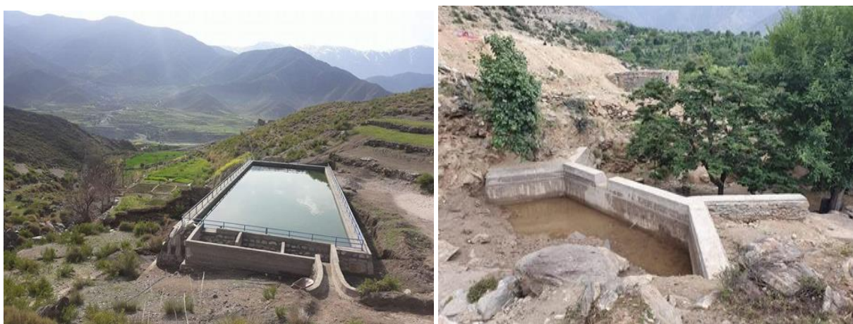
Fig. 2. 1: Rainwater collection from ground surface in Afghanistan
