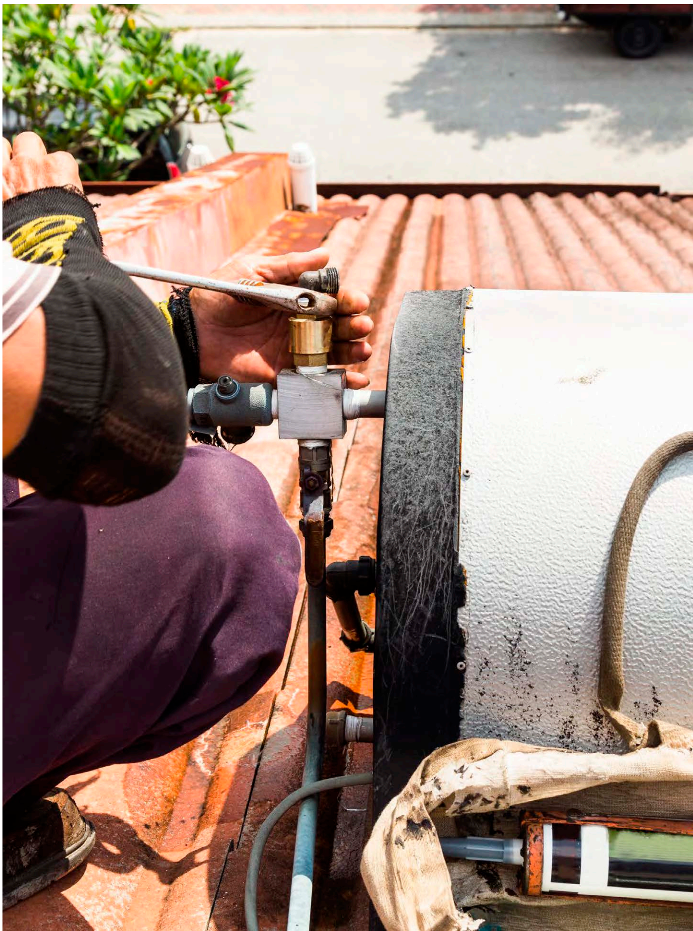
Closeup of worker fixing solar water heater on top of roof during maintenance work. Photo credit: ThamKC/Shutterstock.com
