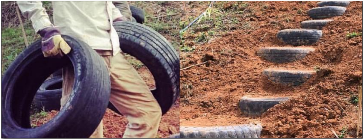
Figure 3.1: Tyre bonding as a means to prevent soil erosion on farms
