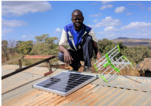
Figure 7: A photo of a man on a rooftop working on a solar PV of a solar home system
