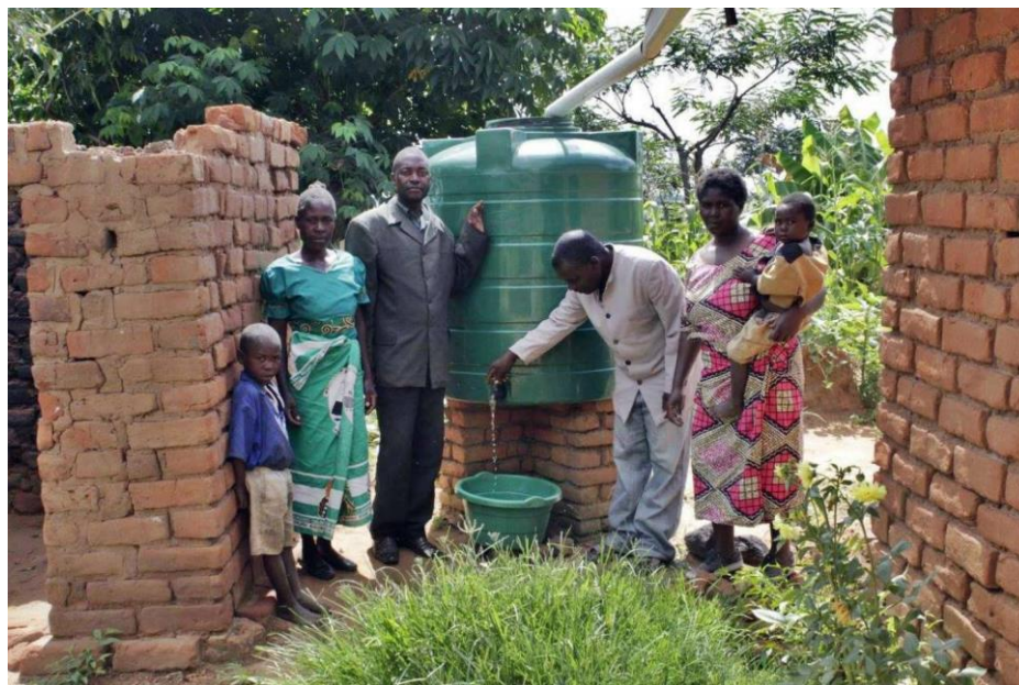
Figure 7: A household in Kamsonga village in Ntchisi District with a rooftop rainwater harvesting system (Source: https://watercharity.com/conclusion-kamsonga-region-rainwater-harvesting-and-well-project-malawi )
