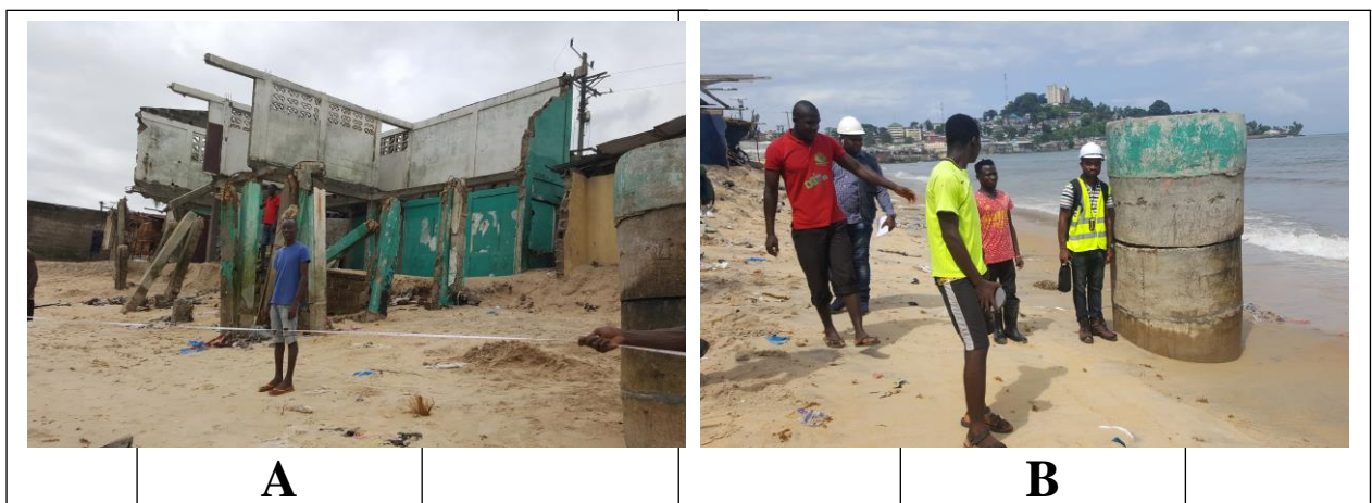
Figure 4: (A), Destruction of properties and (B) - Intrusion of sea/ salt-water into wells; West-point Township; Monrovia – Liberia. Source: Personal; taken June 16, 2019
