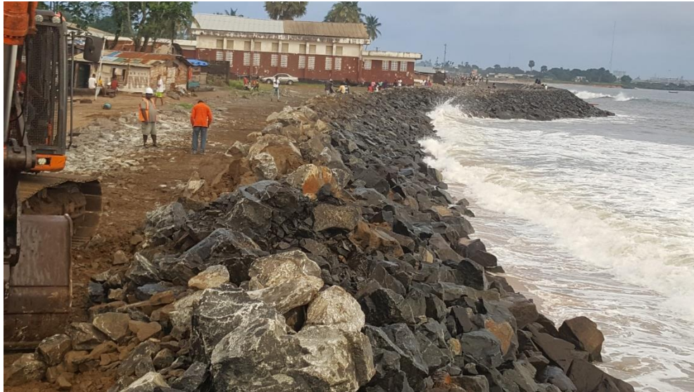
Figure 5: CAP Coastal defence project (Revetment), D-Twe, Kru-Town: Monrovia – Liberia Source: Personal; taken in March of 2019.
