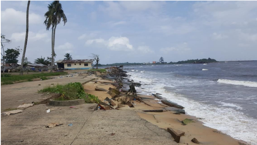
Figure 3: Destruction of Mississippi Street by coastal erosion, Greenville – Sinoe County, Liberia. Source: Personal; taken on June 20, 2019.
