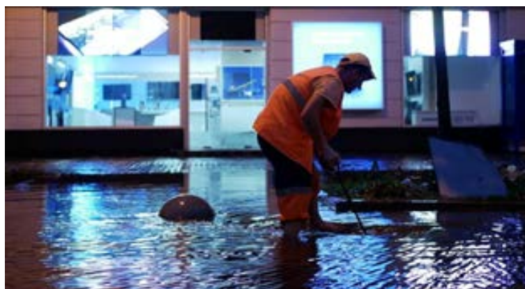
Figure 4.12. Manual cleaning of collectors of municipal drainage rainwater system during flash flood after heavy rainfall in Kyiv, 18 August 2018. Photo by Vladimir Bugaenko.
