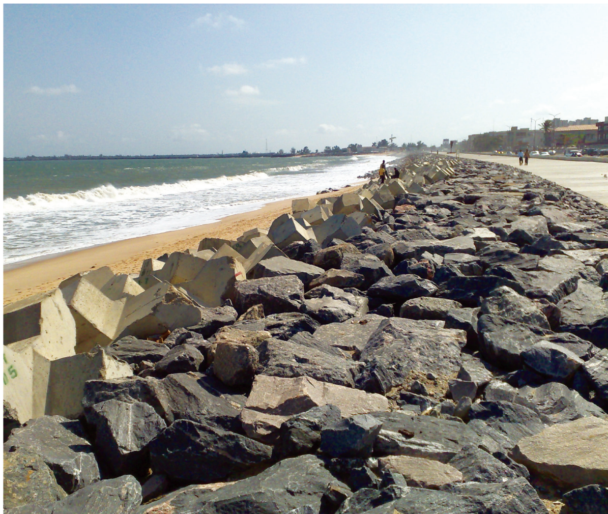
Figure 4.10: Le brise-lames de Bar Beach, Victoria Island, Lagos, Nigeria
