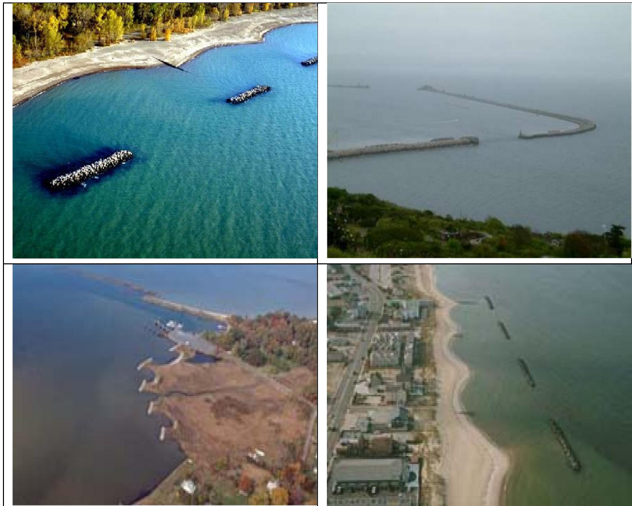
Figure 5: Various Types of Breakwater Systems
