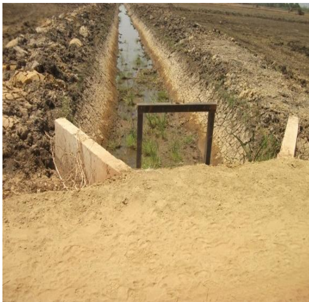
Figure 1a: Primary canal with a gate
