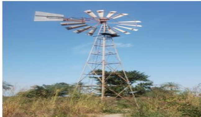
Figure 8: Typical wind pump system
