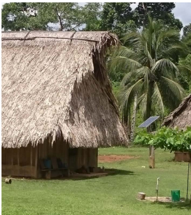
Figure 1: Solar panel installed in Santa Teresa, Toledo District.
