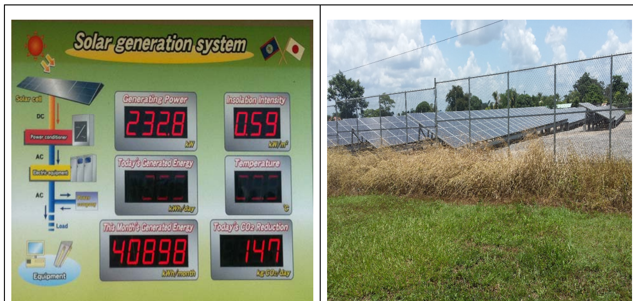
Figure 26: Solar PV On Grid system at the University of Belize central campus
