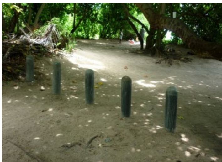
Figure 13. Bollards installed to protect dune at Anse Royale beach.
