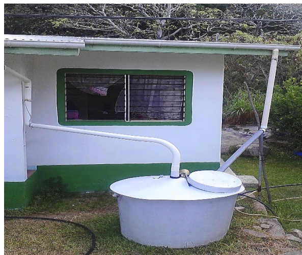
Figure 2. Typical rainwater harvesting system in household in Seychelles with a 500 litre fiberglass rainwater tank.
