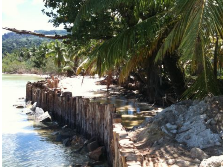
Figure 11. Timber piling to control coastal erosion at Anse Boileau on Mahé.
