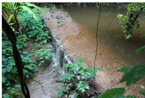
Figure 4. Embankment regulating water flow and increasing water storage on Mahé.
