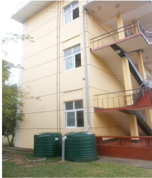
Figure 1. Typical rooftop rainwater harvesting system in a building with 2 x 500 litre polyethylene rainwater tanks.
