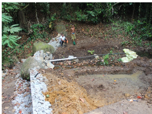
Figure 3. Construction of embankments on Mahé.
