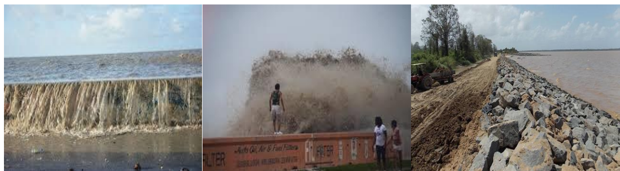
Seawalls and overtopping in Guyana
