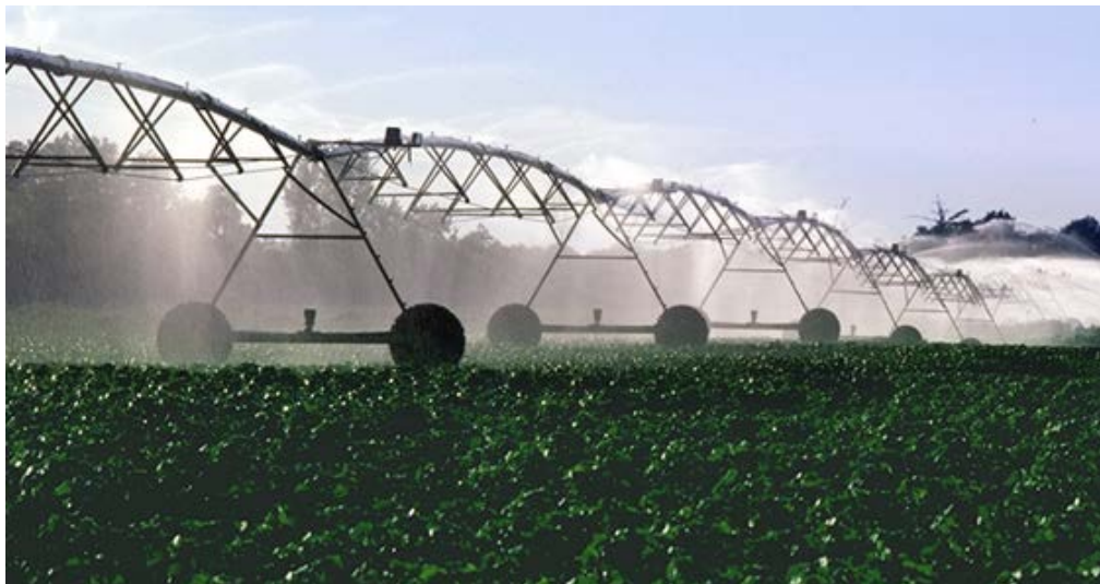
Figure 11: Center Pivot Sprinkler Irrigation System
