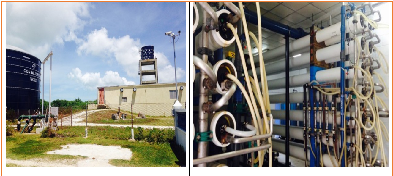
Figure 16: CWBL water storage tank and filters used at the RO Plant in San Pedro
