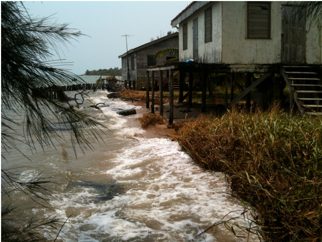
A scene of the intense beach erosion in the Monkey River Community, where the first row of houses has disappeared into the sea. (Source: R. Frutos, June 2016)
