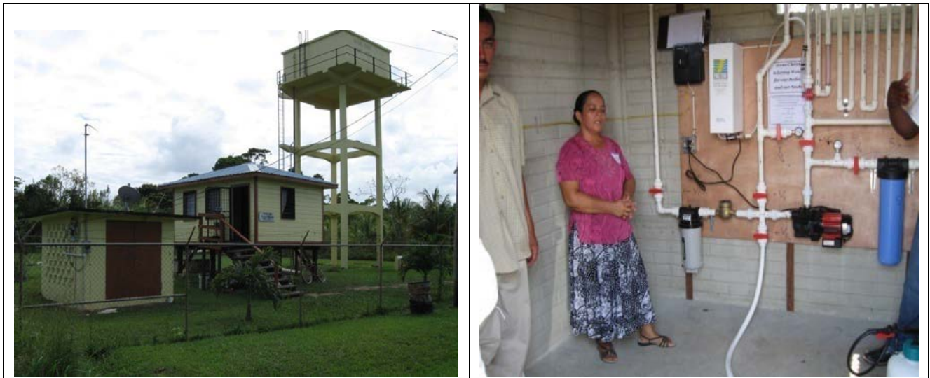
Figure 8: Rural Water System infrastructure and water treatment facility
