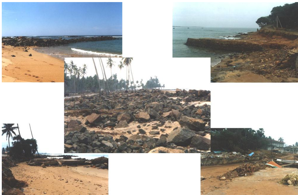
Plate 1: Disturbed revetments & groins in the Southern Coastal belt of Sri Lanka during tsunami
