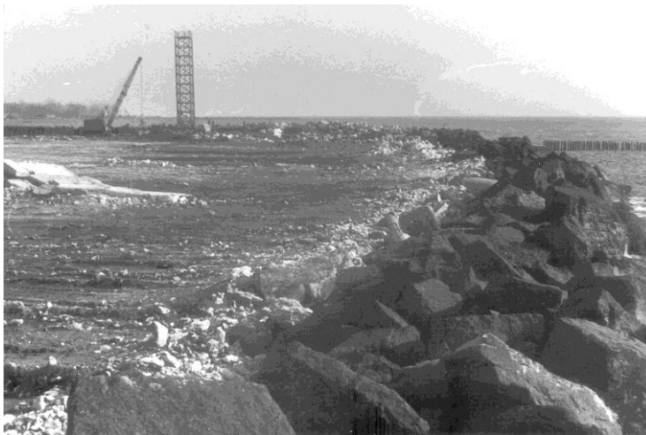
Photo 5. Town Poti, Dike on isle Poti, 1974
