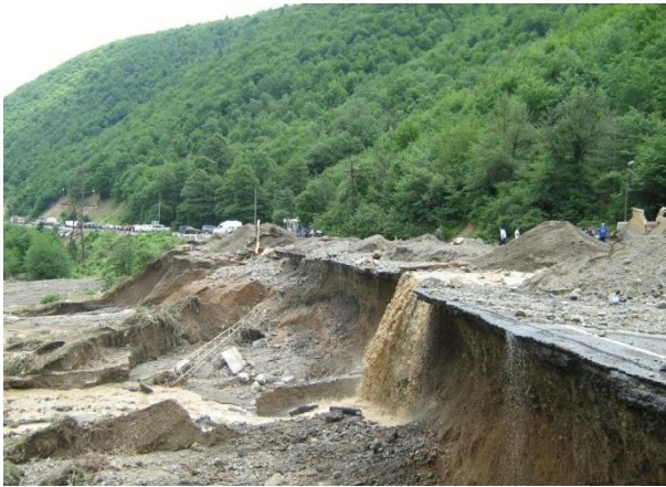
Photo 2. Most recent extreme geological event. 18 June 2011. More than 100 mm rain during two hours were observed on 18 June 2011 at the Rikoti Pass. As a result 6 persons were died, highway infrastructure was destroyed in this segment and more than 1000 housing estates were flooded and damaged by mud stream.
