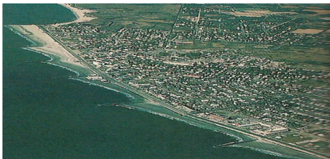
Photo 6. Beach filling process between jetties (in the given case between the capes)
