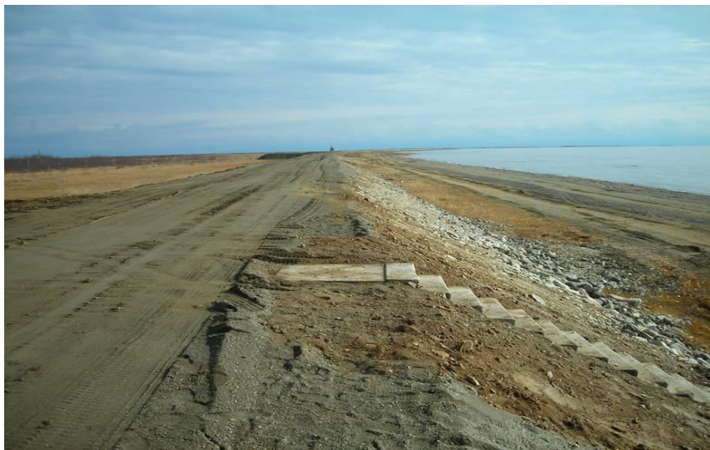
Photo 8. Artificial growing of knolls in width and height
